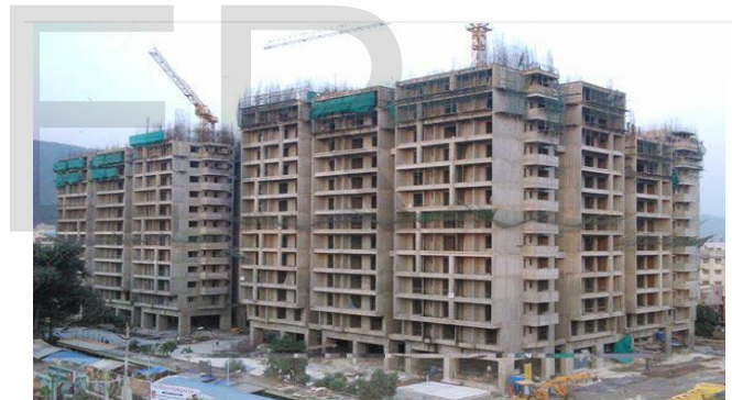
Figure: 8 Oxygen towers, Visakhapatnam, India
