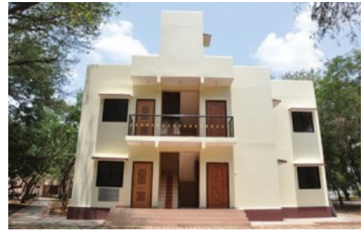
Figure: 7 GFRG residential building, IIT, Chennai
