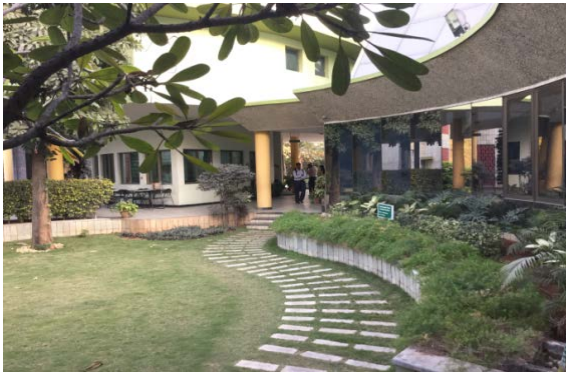
Figure: 11 CII-Sohrabji Godrej Green Business Centre, Hyderabad
